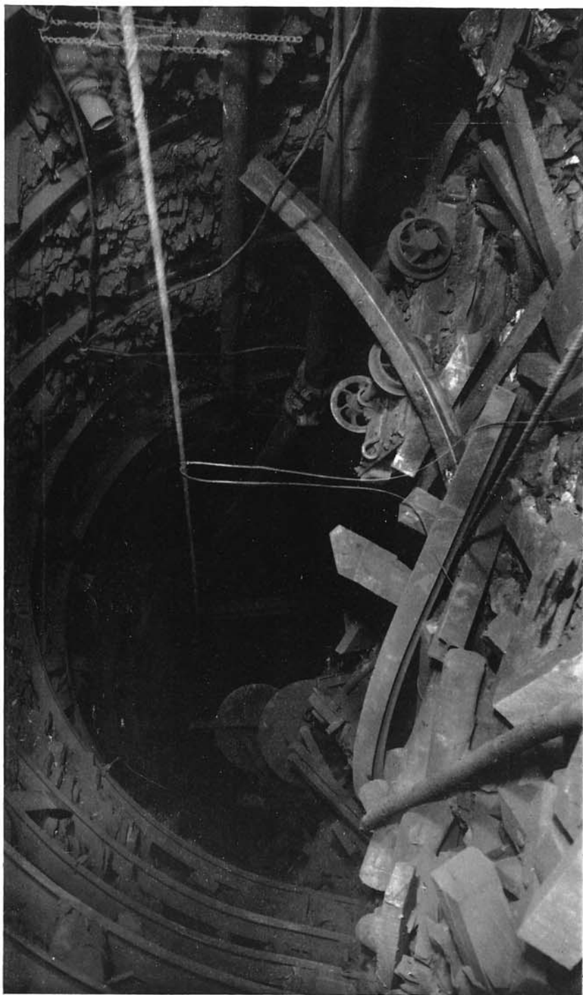
PLATE II. Return gate immediately outbye of haulage return wheel.
